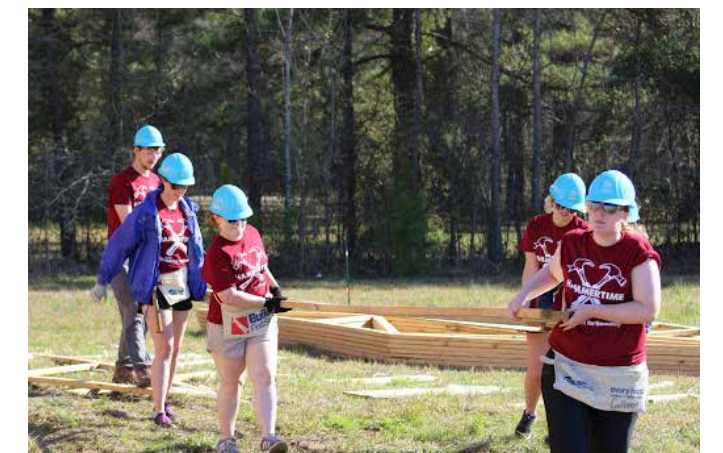
Several habitaters work together to move one of the trusses
