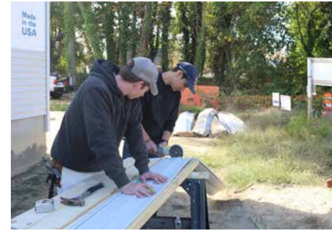
Ryan Mckim '20 and Ben Lammers '20 work together to cut a piece of siding.
