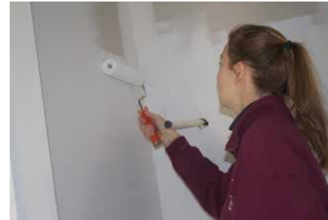
Shannon Thomas ('19) uses a smaller paint roller to paint one of the corner walls
