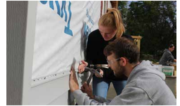
Grace Hazelhurst '23 and Jon Luciani '20 nail in a piece of siding onto the house
