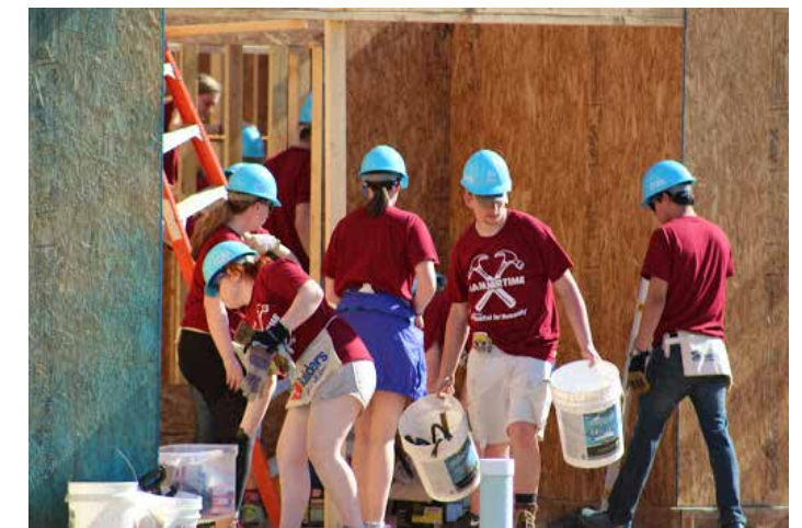
The group begins to lean up after one of the workdays
