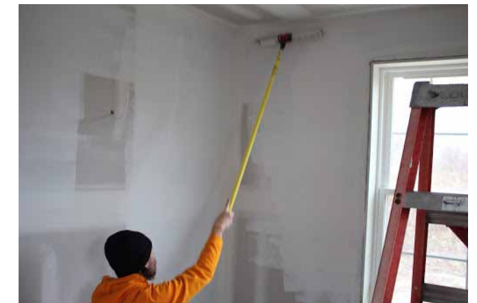
Kyle Bunts ('20) uses a longer paint roller in order to paint the ceiling of one of the rooms
