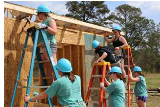
Some team members spot the ladders while others hammer in nails
