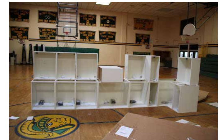
One of the kitchen sets is almost complete
